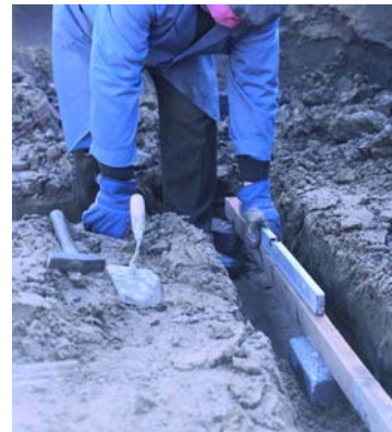
Fig.: Construction aid paving stones
