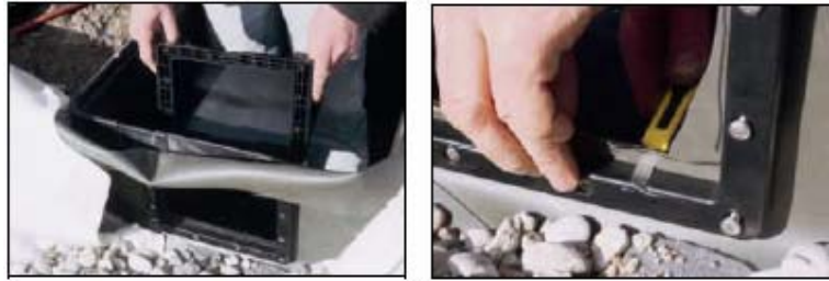
Fig.: Flanging on the skimmer flap
